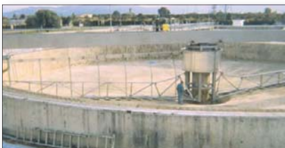
Central Circular Decanting Bridge
