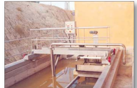
Longitudinal Decanting Bridge
